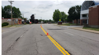
Pavement Marking Project
