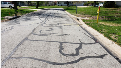
Street Crack Sealing
